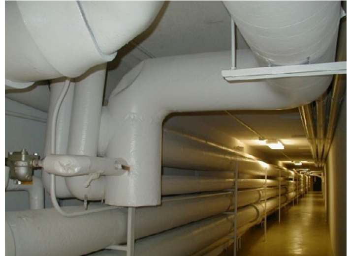
Figure 1: Steam Distribution System
